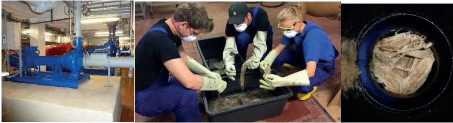
Figure 1 Wastewater pump and analysing clogging material
