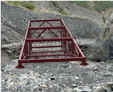
View of the structure before the debris flow passage
