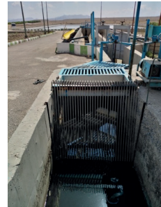
Figure 2 The upstream screens
